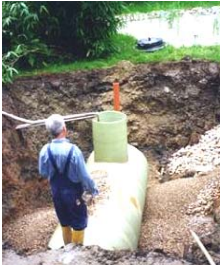
Figure 4.15. Urine tank and constructed wetland for treatment of greywater and leachate from the separation unit in Lambertsühle.
